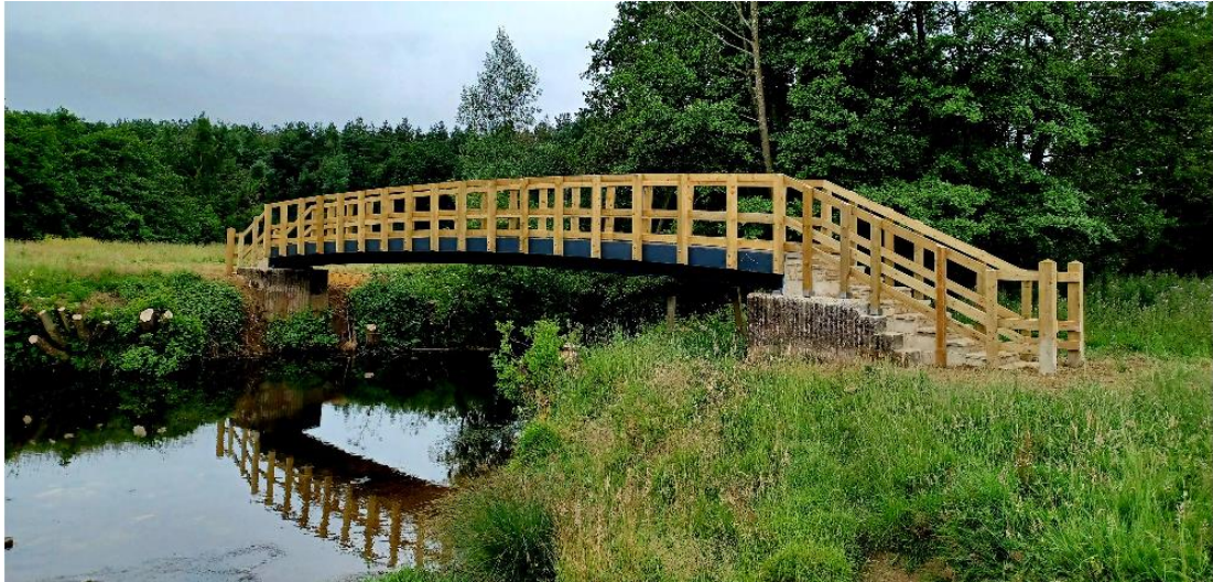
Figure 13 Plump Wood Footbridge, Nunnington
